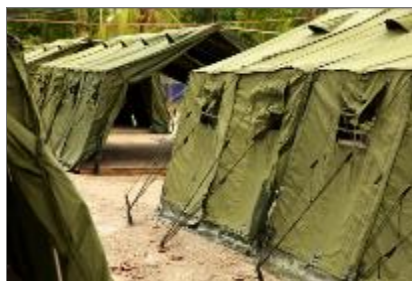
Manus Island regional processing facility Photo Courtesy: DIBP images
